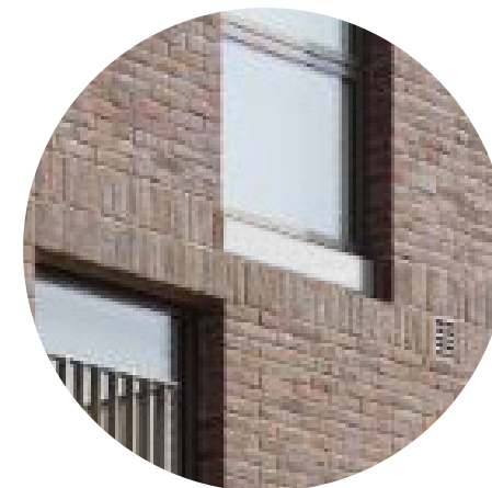
Recessed pre-cast light grey concrete windowsill
