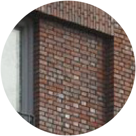
Recessed panels of brickwork
